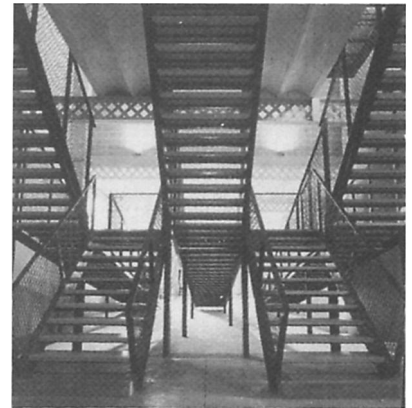
6. La Lluana School, triple stair-ramp
